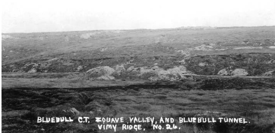
The Blue Bull communication trench was used by the ill-fated nos. 2 and 3 parties to reach No Man's Land at the beginning of the raid.
